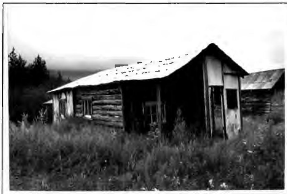
Figure 118. The Jensen/Miller/Stuver Cabin, 1993. The view is looking northeast.
